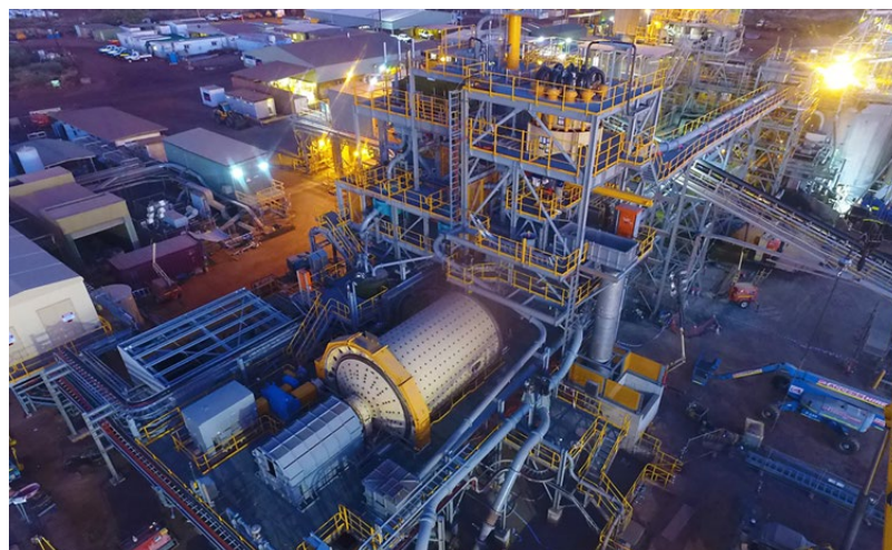
➤ Newmont's Tanami mill in the Northern Territory.
