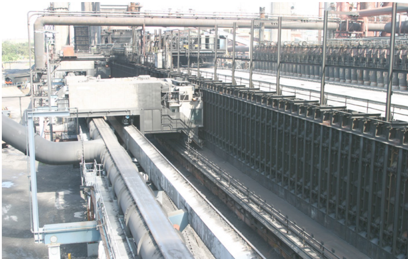
FIGURE 3: A NUMBER OF INDIVIDUAL OVENS MAKE UP A COKE BATTERY
